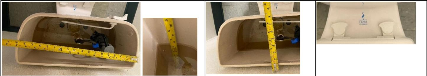
These are helpful to show the tank width, front to back “depth” and water level depth. The logo is also often helpful because some logos are indicative of a date of manufacture. \*Photos are a sample only. This tank is actually 1.6 gpf
